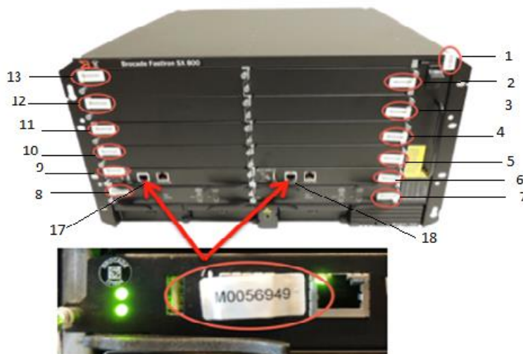
Figure 84 - SX800 (containing SX-FI-ZMR-XL management modules and SX-FISF Switch Fabric modules) - Front view with tamper evident label security seals
