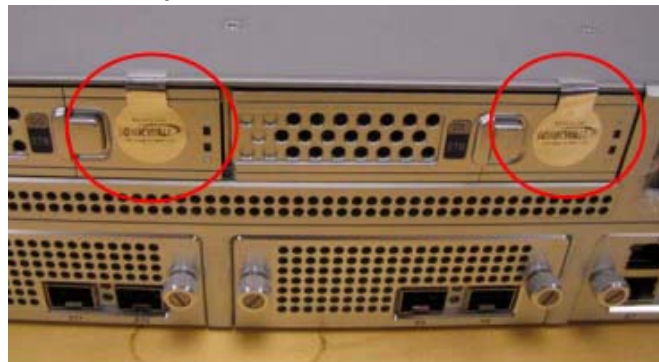
Figure 8 –SRA CBCSPs and EX9000 Tamper Seals #6 and #7 - Front Drive Bays
