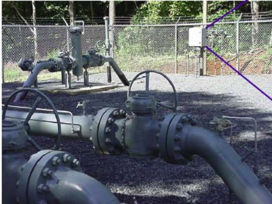
Remote Terminal Unit (RTU)
