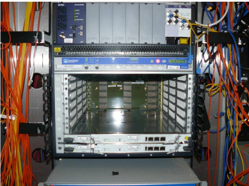
Figure 8. MX960 with Routing Engine
